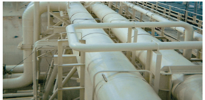
GRP Cladding Erection
