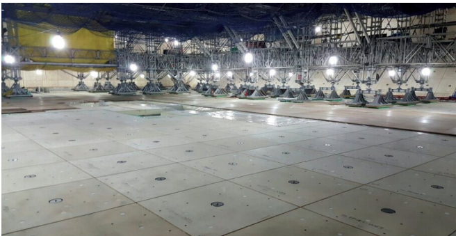
Erected KC-1 Insulation Panel
