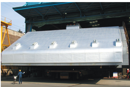
Upper block Insulation
